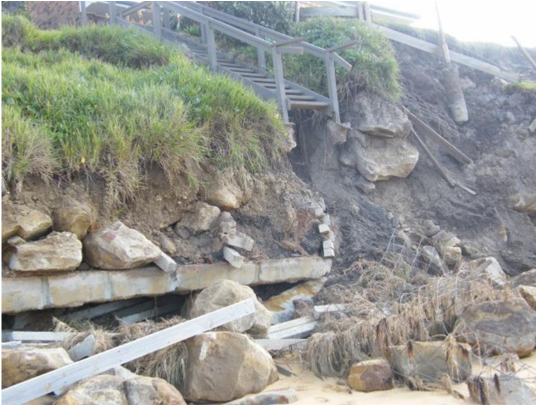
Plate 3 – Eroded escarpment on Wamberal Beach with collapsing structures, voids and suspended rock posed an immediate hazard following June 2016 storms. Photo: Coastal Environment, June 15th 2016.
