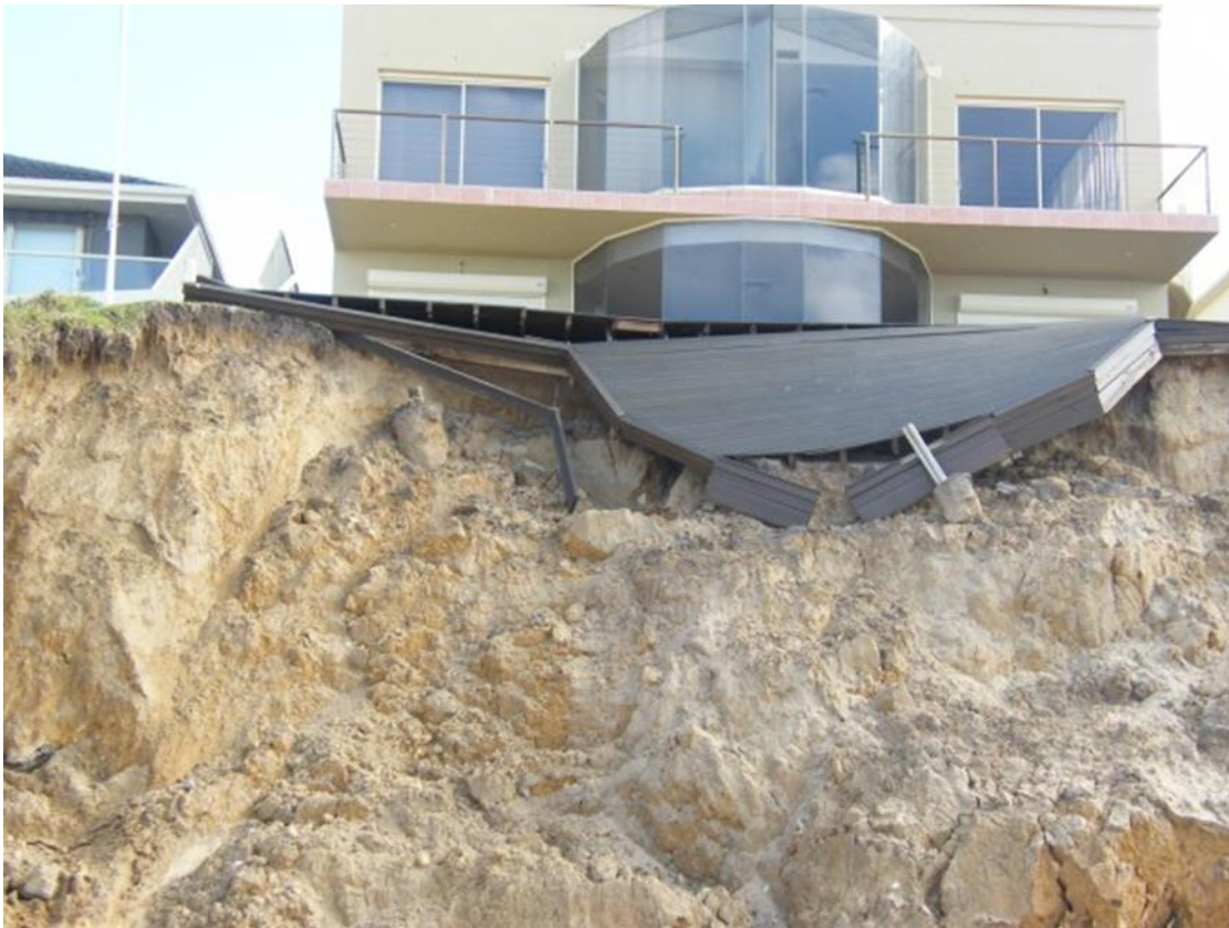
Plate 2 – Five metre high storm erosion escarpment undermined fencing and timber deck on Wamberal Beach. Photo: Coastal Environment, June 15th 2016.
