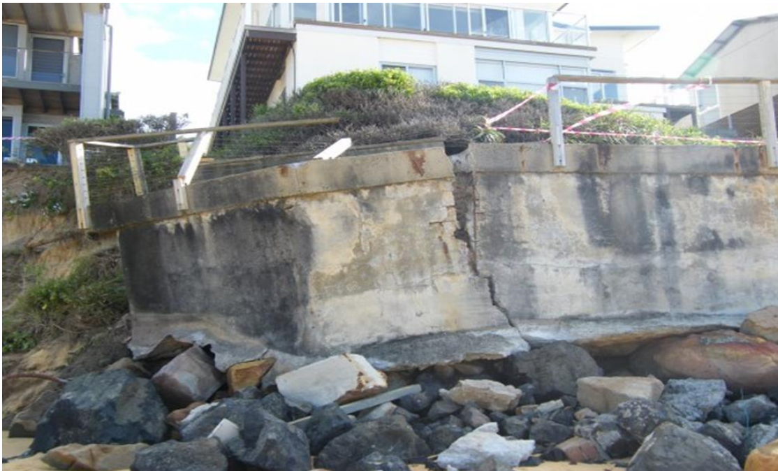
Plate 1 – Concrete seawall on Wamberal Beach undermined and damaged following June 2016 storms Photo: Coastal Environment, June 15 th 2016.
