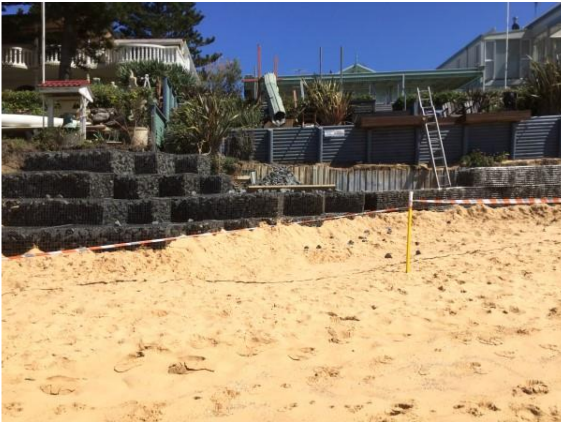
Plate 5 - Gabion revetment under construction at Wamberal Beach following June 2016 storm erosion.
